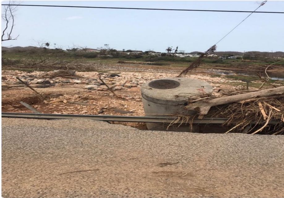
Manati Trunk Sewer
